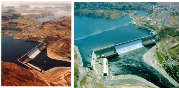
Figure 2 Grand Coulee hydroelectric Plant
